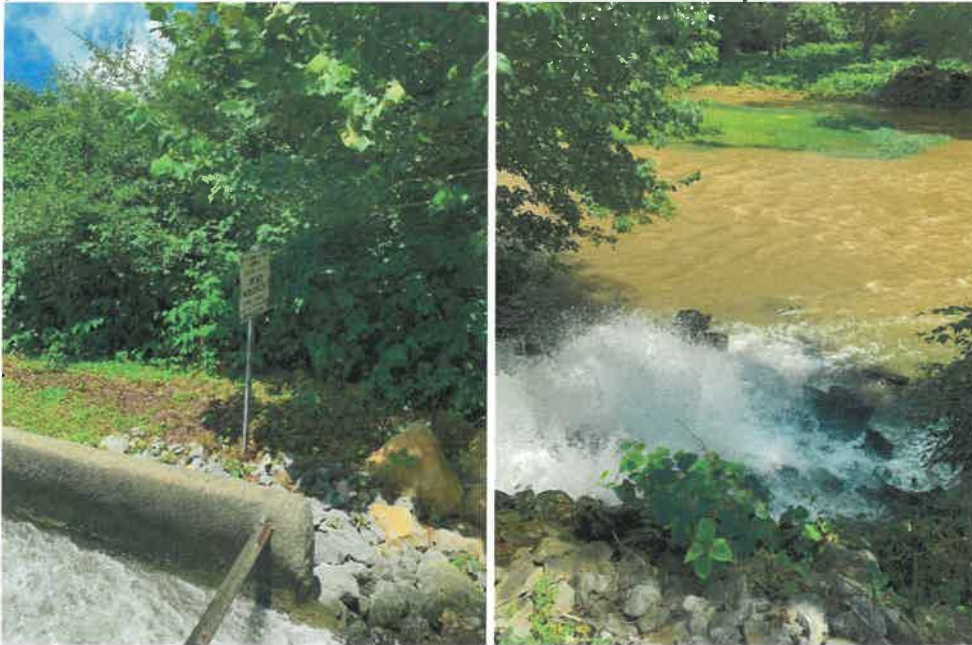
Lagoon Outlet 001 outfall and marker (no concerns noted)
